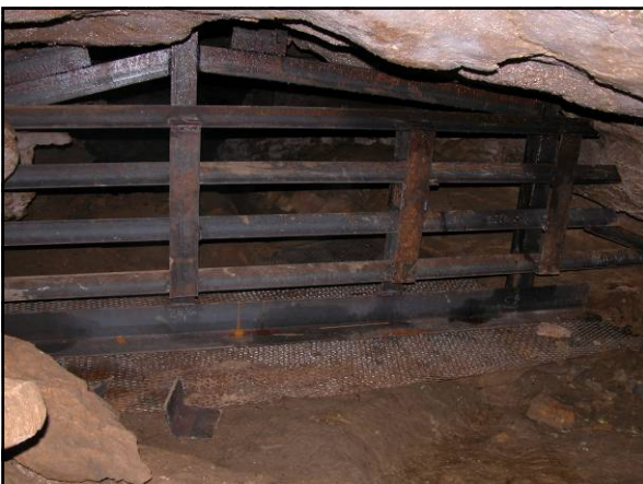
Completed cave gate. Photo courtesy of USFWS.
